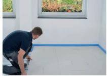
Press the element down firmly. The adhesive will swell out of the joints slightly.
