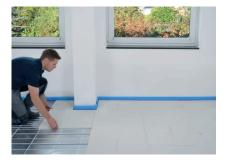
Cut individual cut-outs to size and adhere these, too, into the tongue and groove connections.
