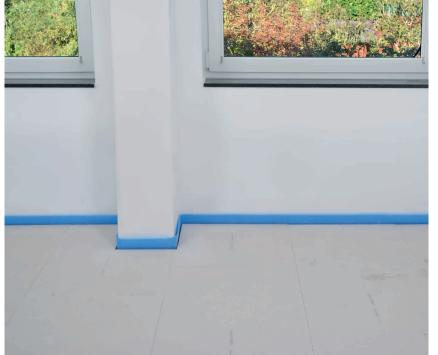
After a drying period of 24 hours, the excess adhesive can be pushed off.
