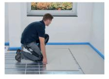
Push the element together in the tongue and groove connection.
