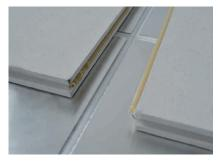
Add adhesive string to the underside of the groove as well as the upper side of the tongue. (approx. 10 m²/cartridge).
