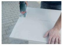
Shorten the last element of each row to length (e.g. using a Diamaster circular saw blade or a Jigsaw blade T141 HM, Bosch).
