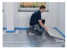
Start laying in the left-hand corner of the room. Do not press the edge insulation strips together.
